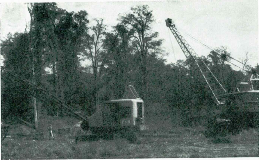
Fig. 13. Mechanization project Shanka. Two draglines of the Dragline-dredging operation. Adola district
